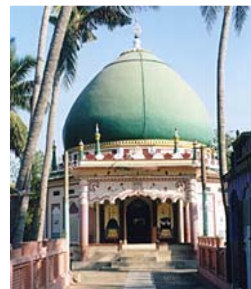
Fig 10.9: Quadam-i-Rasool at Cuttack
