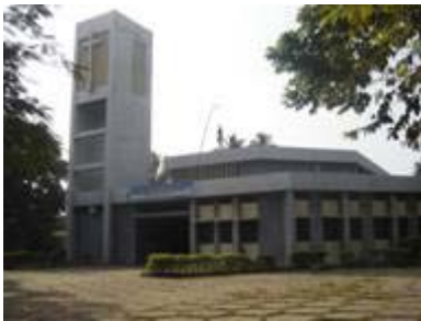
Fig 11.26: Church in Cantonment Area
