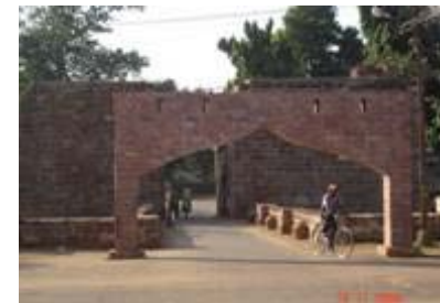
Fig 11.14: Barabati Fort Entrance Gate
