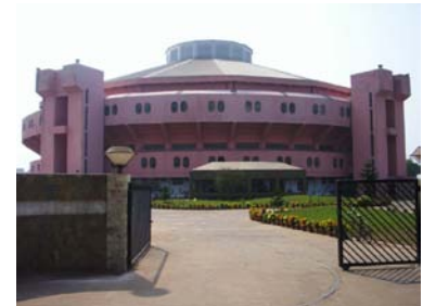
Fig 10.3: Indoor Stadium at Cuttack
