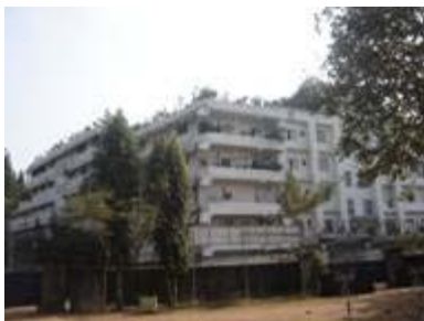
Fig 11.27: Cambridge School- construction of high rise buildings
