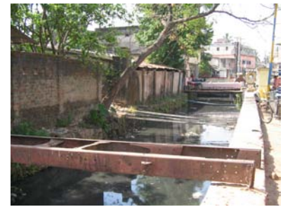
Fig. 12.8: Open drains near roadsides in Cuttack
