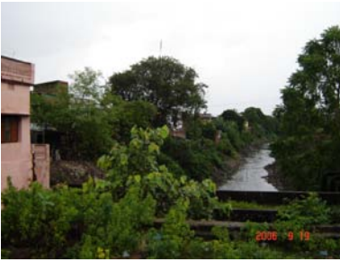
Fig 8.13: Disposal of Main Drain into Kathajodi River, a view at Khannagar
