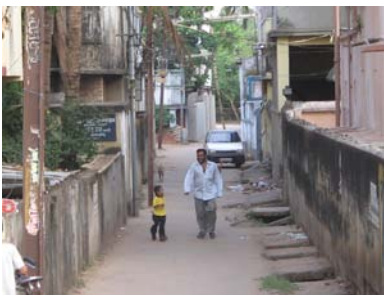
Fig 12.2: Narrow lanes with houses joined to each other without setbacks increases the vulnerability during fire
