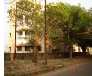
Fig 7.1: LIC Housing at Bidanasi Sector, Cuttack
